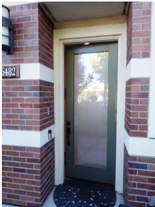
Front door entrance appeared serviceable
